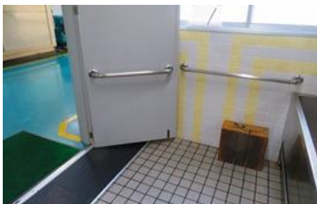
Barrier-free for preventing tripping and falling (Yana Factory)
