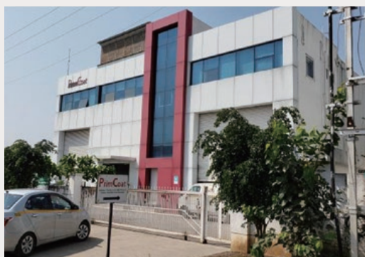
Coating hub in India
