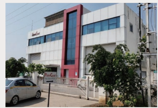
Coating hub in India
